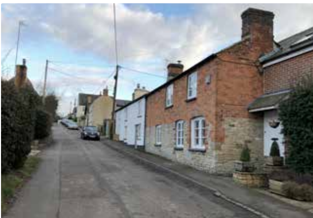
Mixture of building materials along Freehold Street
