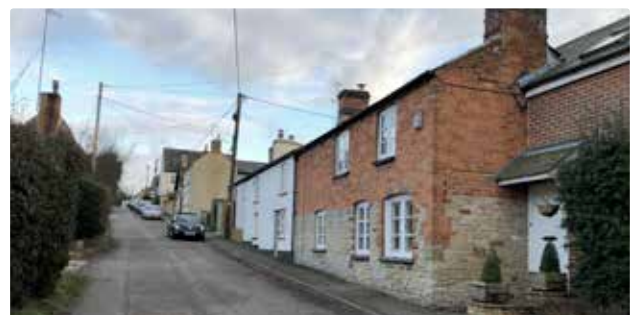
Mixture of building materials along Freehold Street
