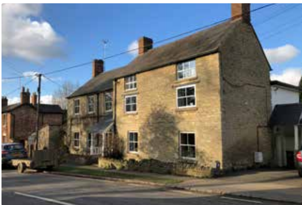
Cottages Station Road
