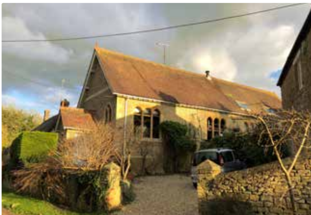
Methodist chapel now house
